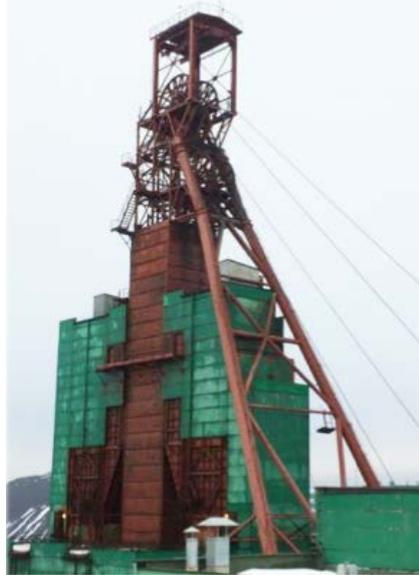
The single-layer double drum with a diameter of 5 m lifts a load to a height of 480 m in around 11m/s. After 244,000 cycles, the rope was removed, and the areas exposed to the greatest stress during operation in the mine were examined in the lab. Neither the loss of profile nor the wear and corrosion on the inner side of the rope were significant as yet. The breaking strength measured was, despite the high number of load cycles, still above the minimum breaking strength guaranteed at delivery.
